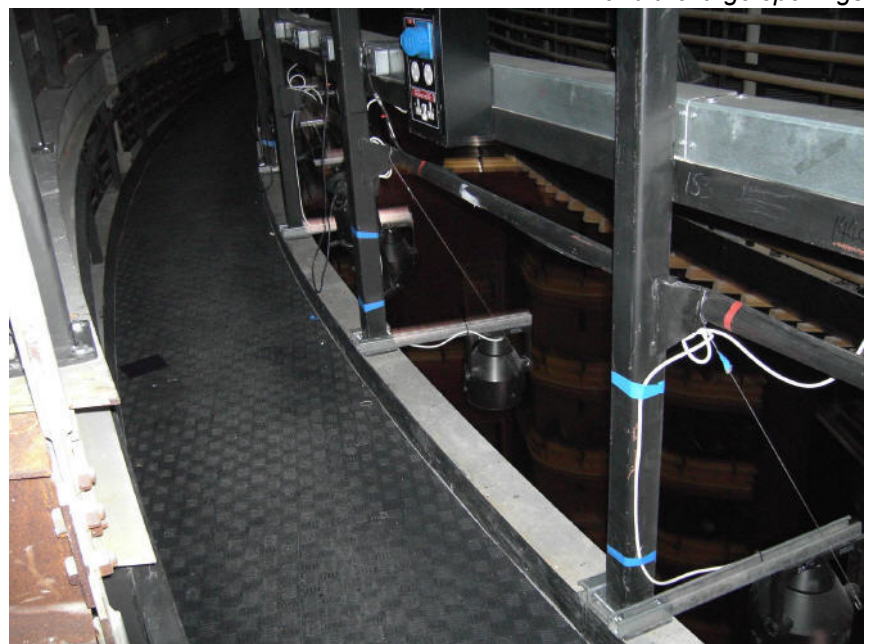
Auditorium lighting bridge showing the lighting rail and the large openings
